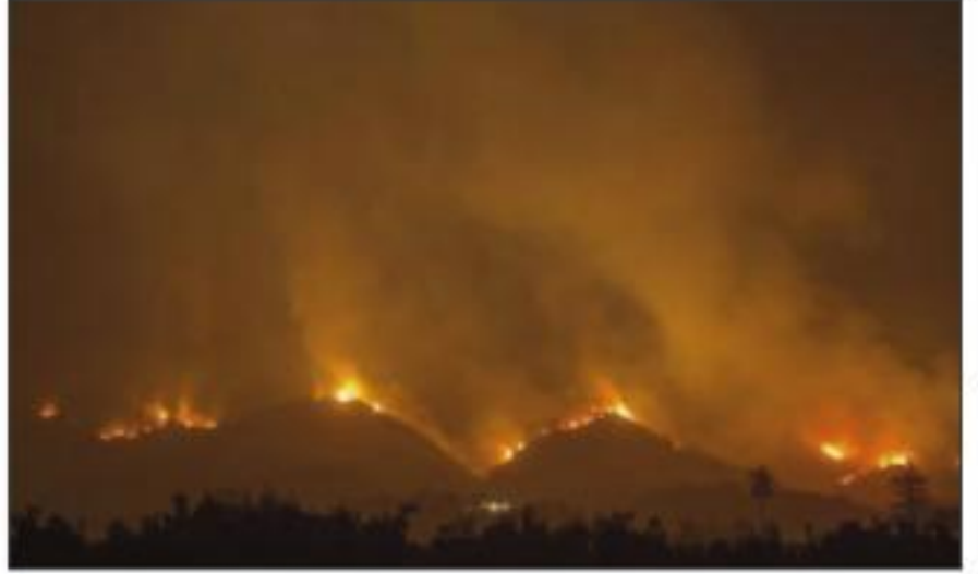
Wildfire engulfs power plant in Turkey
